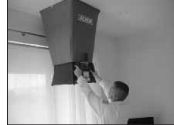
Air flow testing.
